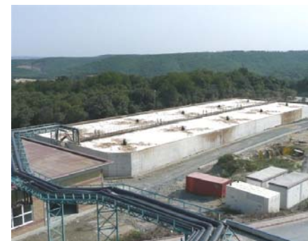
Membrane building (L) aerobic tank 90 x 30m
