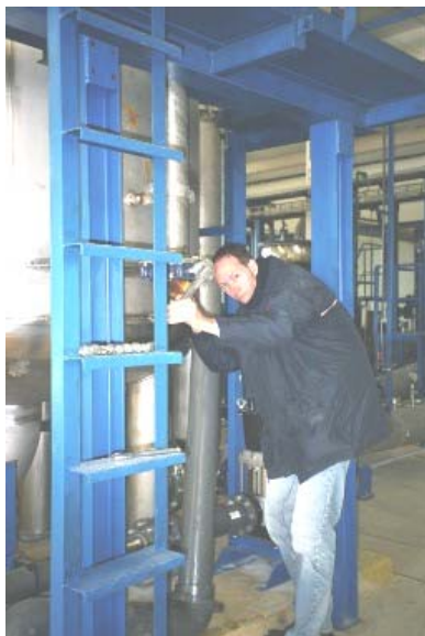
Dismantling PVC pipe under valve
