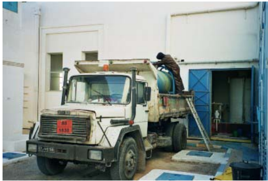
95% sulphuric acid supply by sand truck
