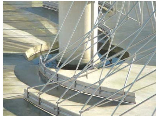
Cone of a Clarifier
