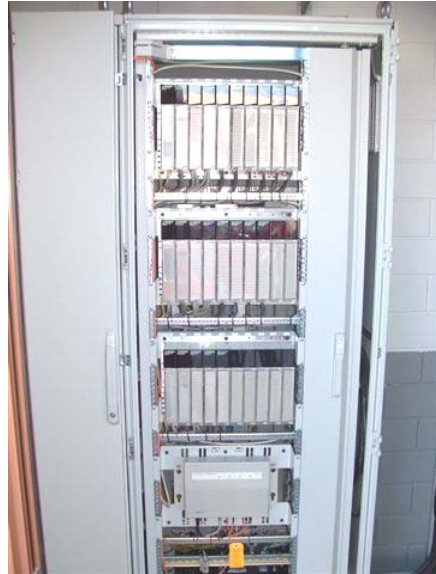
The Smallest of 5 PLC's (HP has app. 8500 IO's)
